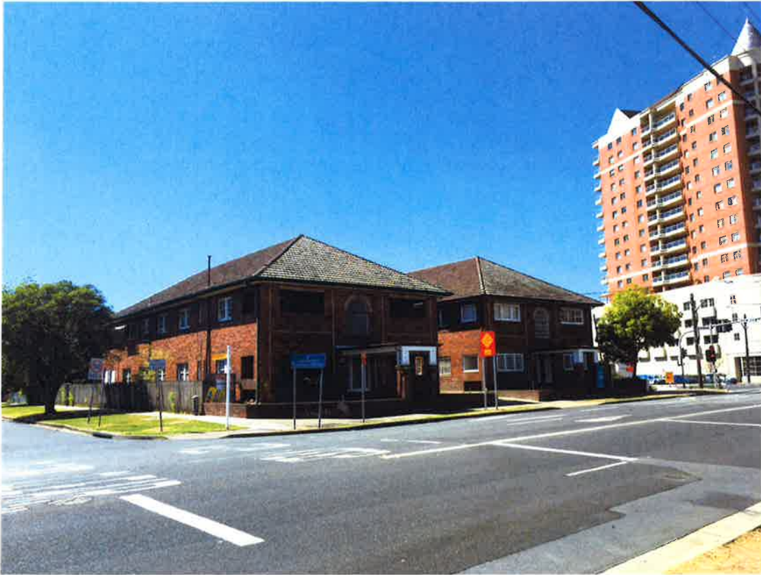
Figure 5: View of site from Albert Road facing north
