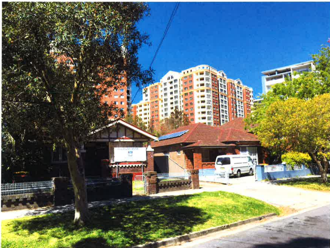
Figure 10: View of existing buildings at 4 and 6 Pilgrim Avenue facing south-east
